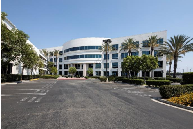
Office Exterior Facade
